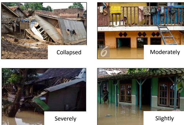
Figure 5. Images and level of damage classification
